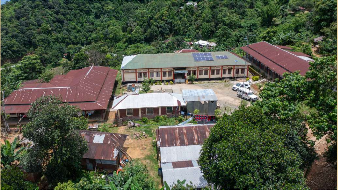
A view of PHC Oniamlong which was solar powered along with an energy efficiency drive providing constant and reliable access to health care
