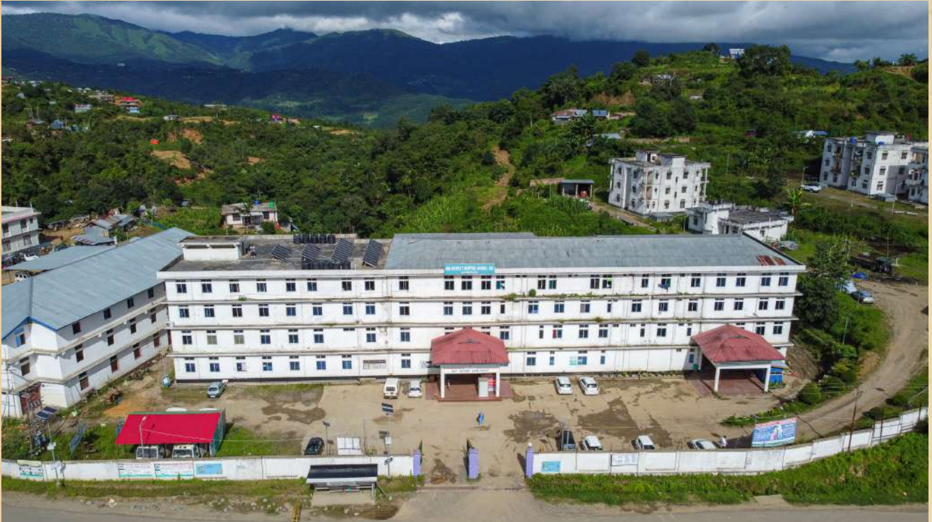
A view of District Hospital Ukhrul which was solar powered along with an energy efficiency drive providing constant and reliable access to health care
