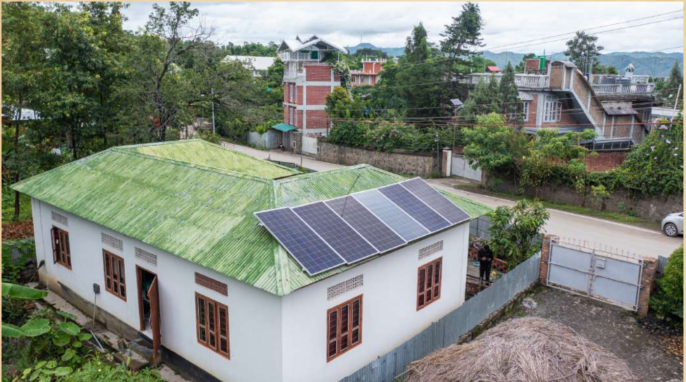
A view of HWC Pearsonmun which was solar powered along with an energy efficiency drive providing constant and reliable access to health care
