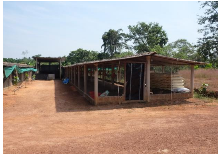
-fig 2. The exterior housing of the broiler farm indicated in fig 1. The building was made by local fabricators. Materials used would have included stone, sand, cement and wood for the structure. Corrugated roofing and asbestos for insulation and rainproofing.
