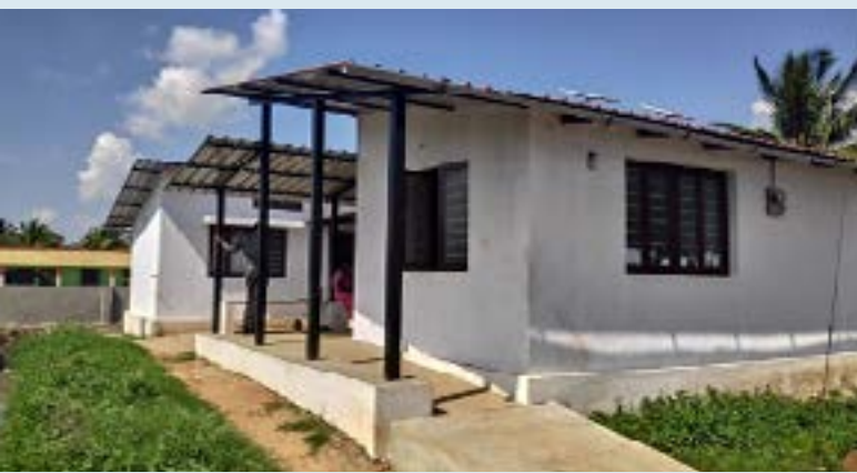
YK Mole Sub Centre designed to ensure thermal comfort for the patients and the health care staff, and reduce energy consumption; ANM Bhagya administering a patient at the YK Mole sub-centre, Gumballi, Karnataka.
