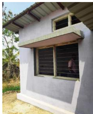
Ventilators and air gaps in the roof for hot air to escape
