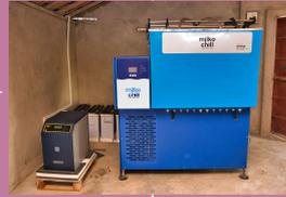
Mini collection center with solar milk cooling solution
