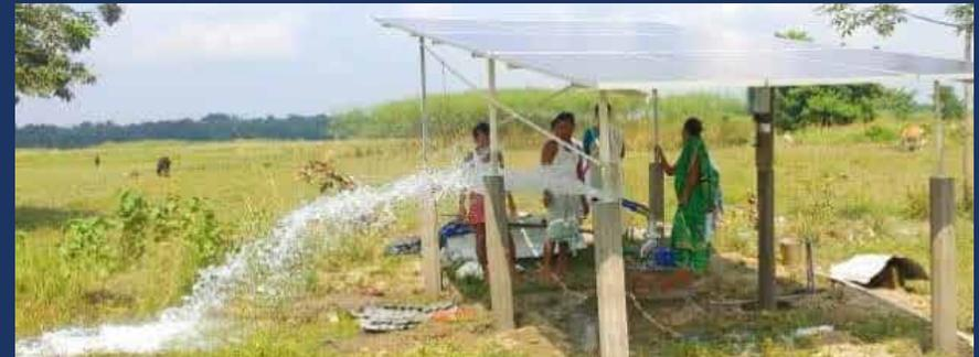
The operation of solar powered pumps is more economical mainly due to lower operation and maintenance costs and has less environmental impact. These can be surface or submersible in nature from 0.5 to 10HP
