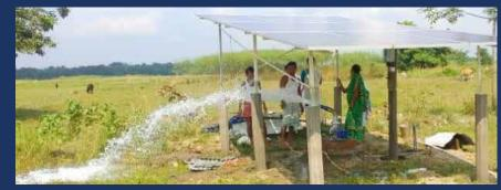
The operation of solar powered pumps is more economical mainly due to lower operation and maintenance costs and has less environmental impact. These can be surface or submersible in nature from 0.5 to 10HP
