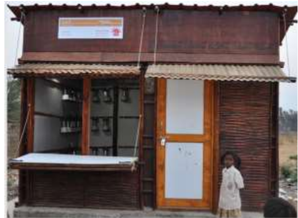
2. INTEGRATED ENERGY CENTER
