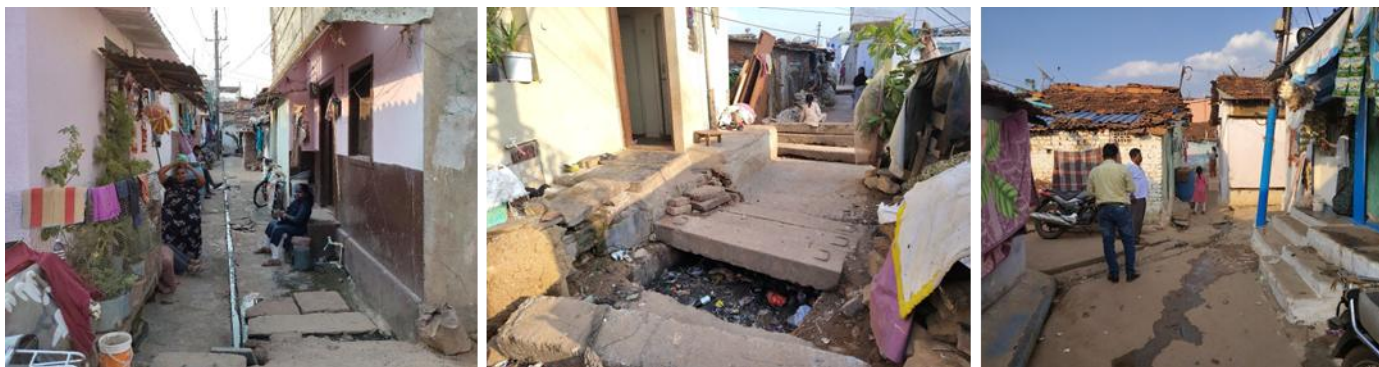
Figure 33 Narrow alleys and encroached natural drains in Jannath Nagar; existing artificial stormwater drains are inadequate during heavy rains.
