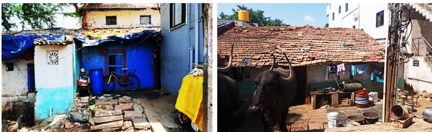
Figure 50 Kutchha houses covered with tarpaulin sheets to protect roofs from weather damage
