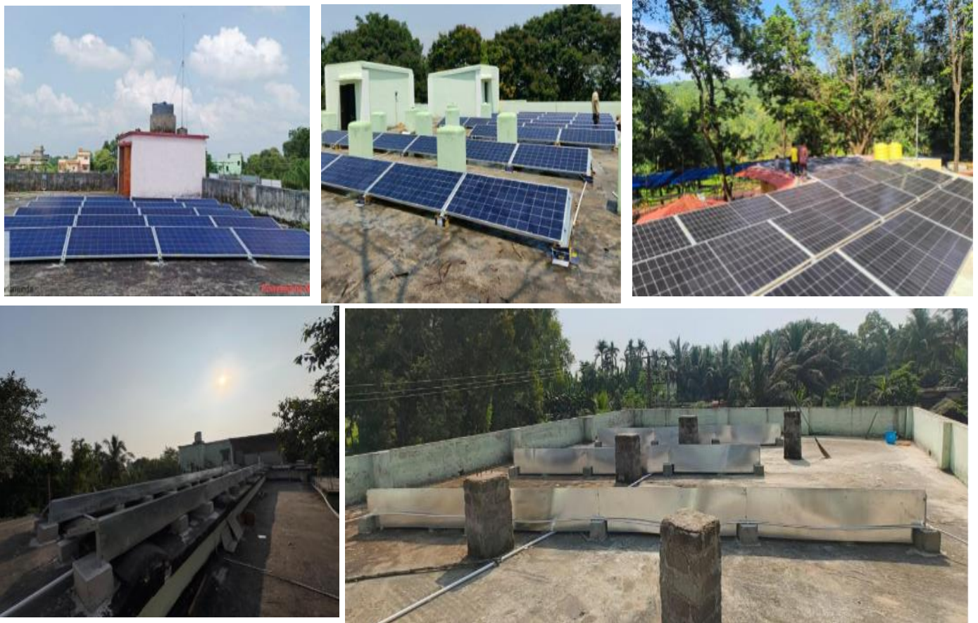
Figure 1: Examples of climate-resilient RCC rooftop solar MMS installations demonstrating low-elevation landscape mounting, optimal tilt, multi-point clamping, wind deflectors, triangular support structures, ventilation and drainage clearance, anodised aluminium members, secure anchoring, and ballast block reinforcement for high-wind and cyclone-prone regions.
